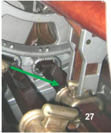
High current marks at contact 27, phase W
