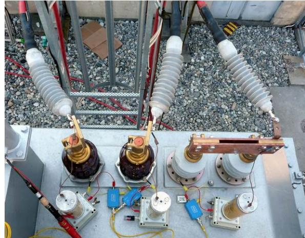
Example for the use of coupling capacitors where bushing connectors without measuring taps were installed at the low voltage terminals.
