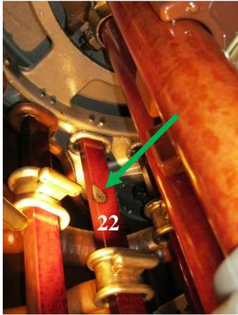
Carbonised track on the insulating rod
