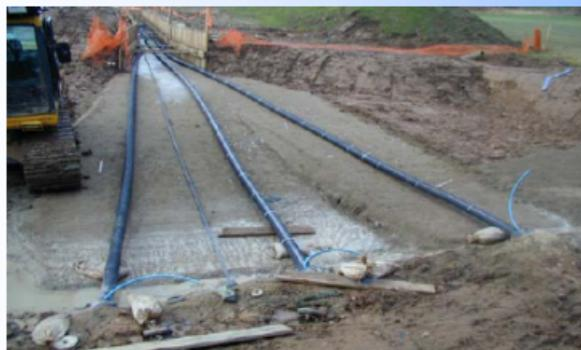
Cable spacing increased as cable enter duct
