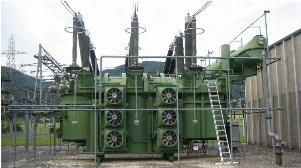
**Figure 10:** Phase shifting transformer (400 MVA, 400/220/49 kV)
