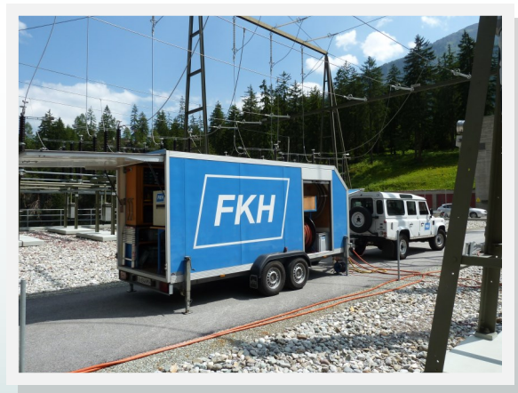
Mobile supply source to generate the experimental ground fault current
