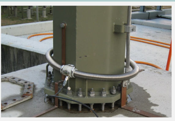
Rogowski coil to measure ground currents in pylons
