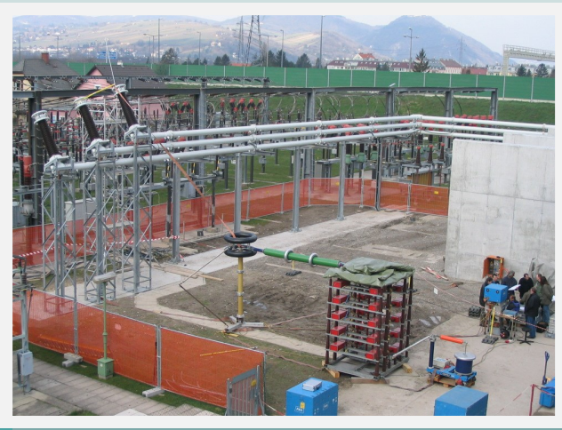
Test on a 123 kV GIS with oscillatory lightning surge
