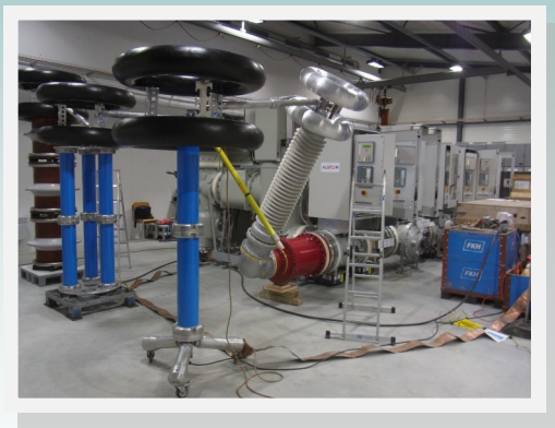
GIS test setup on a 123 kV system
