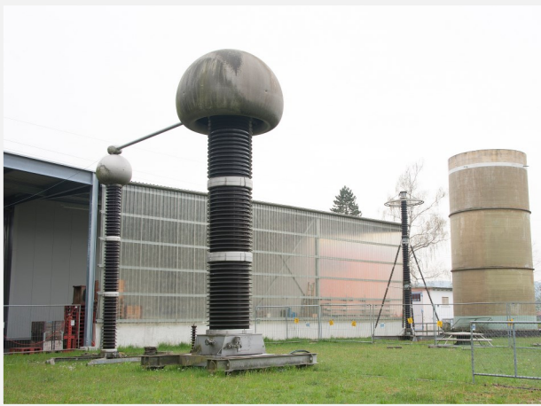
1000 kV test transformer at the Däniken Experimental Station
