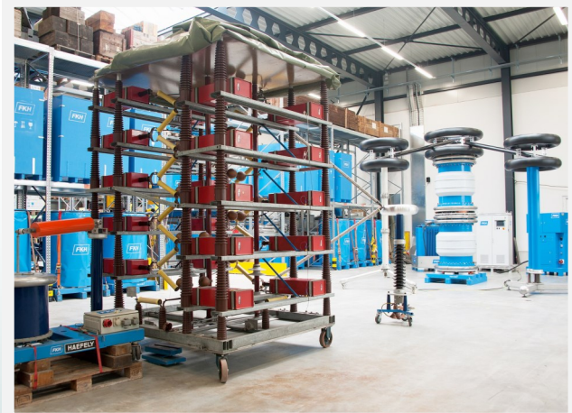
Mobile testing equipment: impulse generator, series resonance test system
