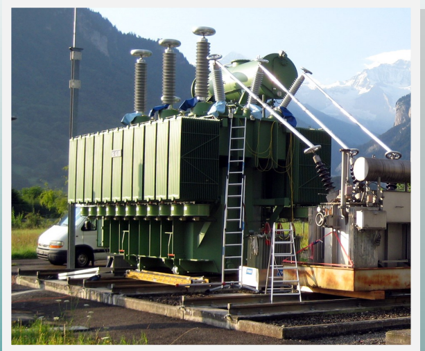
Excitation of a grid interconnection transformer for the partial discharge measurement in a substation
