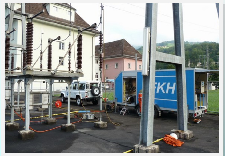
Grounding measurement system: feeding a test ground fault current into an overhead line in a substation
