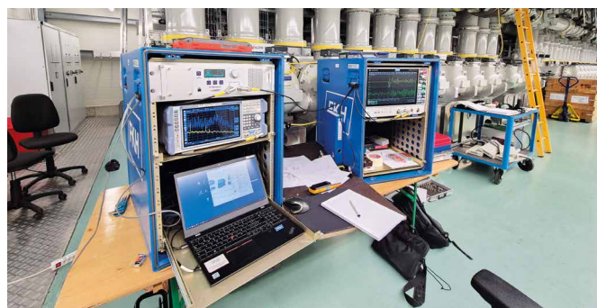
Figure 10: UHF partial discharge test station with multiplexer, spectrum analyser and oscilloscope
