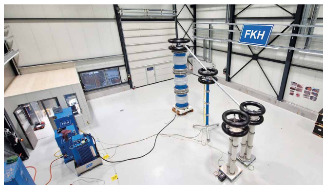
Figure 2: Series resonance system in the large test laboratory
