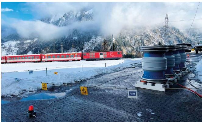
Figure 1: Cable testing using series resonance reactors
